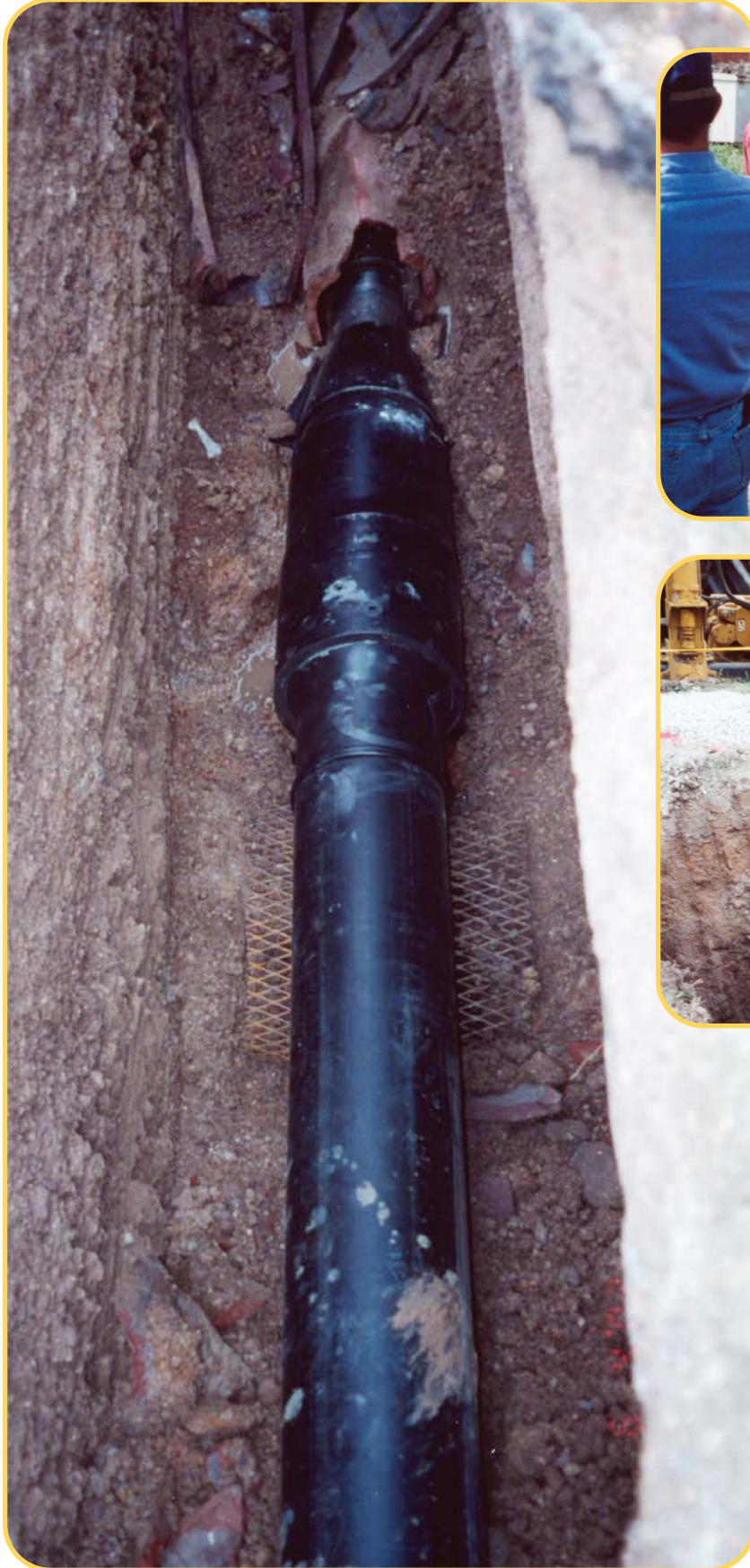
Left: 865' burst begins. Top right: Shoestring crew watches as first 515' is pulled into place. Bottom right: Exiting first 515' burst.
