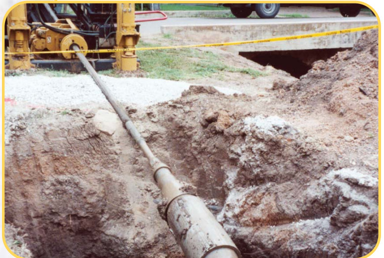
Left: 865' burst begins. Top right: Shoestring crew watches as first 515' is pulled into place. Bottom right: Exiting first 515' burst.
