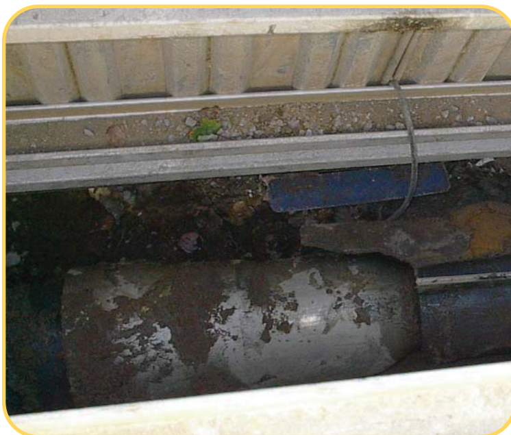
Above: Beginning to pull in the new 12" pipe. Inset: Marvin Sailor (Vermeer of Kentucky), drilling out through the old water main. Top left: Slicing through a huge cast iron bell. Bottom left: The end of the line.
