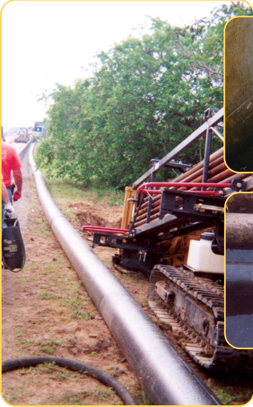
Above: Setting up for the fifth pull of the job. 380' of HDPE is sitting next to the drill for the following pull.
