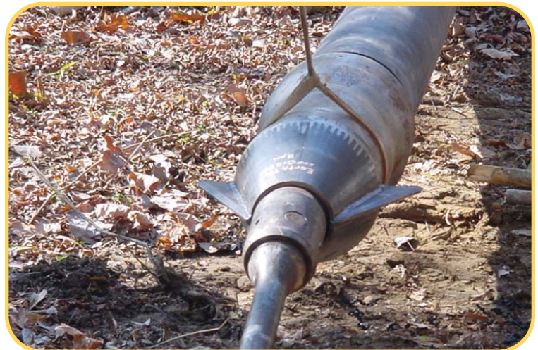
Top: Looking down the line, from the drill set up location. The entry manhole is visible in the distance. Middle: This above ground manhole is the entry point to the first 380' burst segment. Bottom: The business end of the Impactor with starter rod attached. The cutting blades are a new test configuration.
