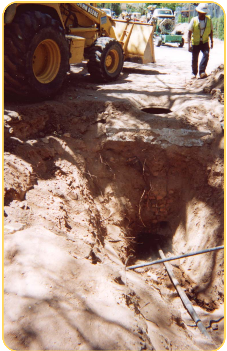
Left: Access hole for D33x44 drill rods to the backside of the exit manhole. Right: Drill rods pushed through existing 6" line.
