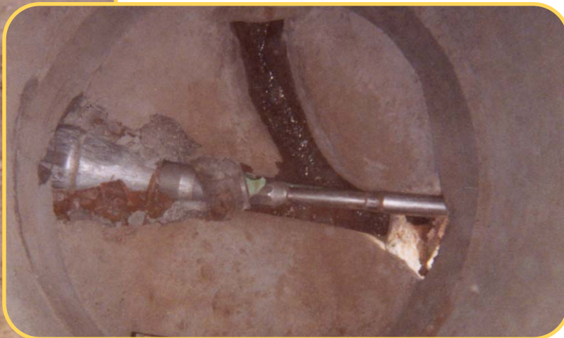
Left: HDPE installed through existing 6" VCP line. Top right: The Air Impactor entering the old pipe under an exposed 1 1/4" gas line utility. Above: The Air Impactor arriving at the exit manhole prior to extraction.
