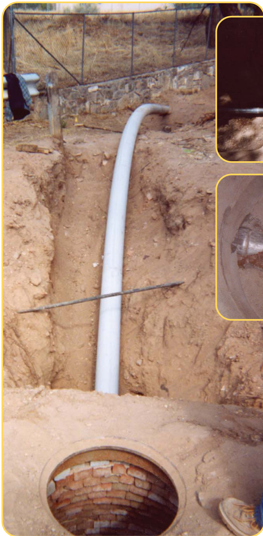
Left: HDPE installed through existing 6" VCP line. Top right: The Air Impactor entering the old pipe under an exposed 1 1/4" gas line utility. Above: The Air Impactor arriving at the exit manhole prior to extraction.
