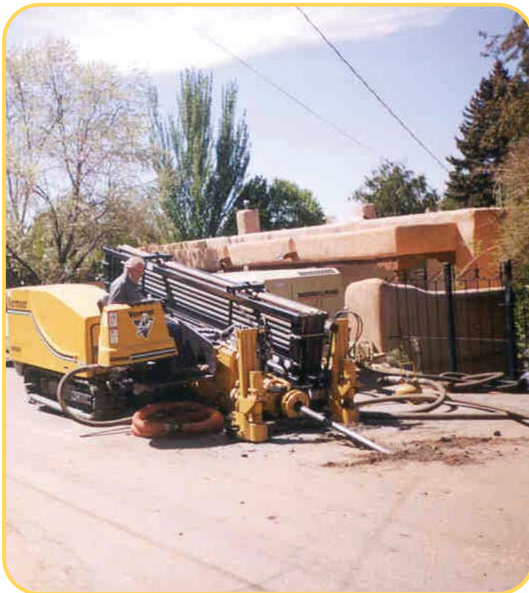
Left: Access hole for D33x44 drill rods to the backside of the exit manhole. Right: Drill rods pushed through existing 6" line.
