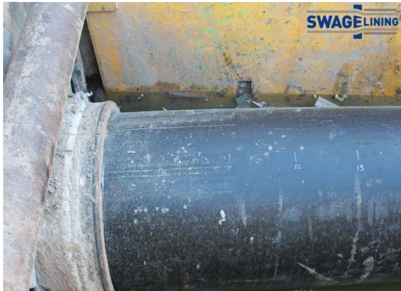
Figure 6: Tight compressive fit of HDPE after reversion.
