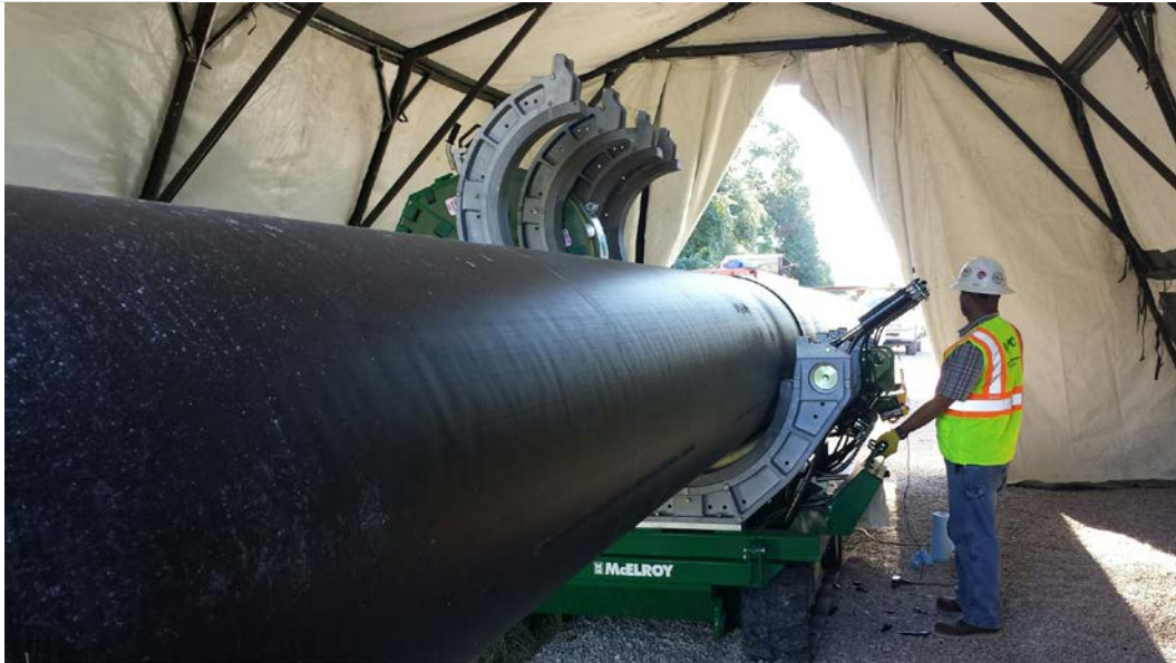
Figure 5: McElroy fusion machine welding 30-inch HDPE within a tent.
