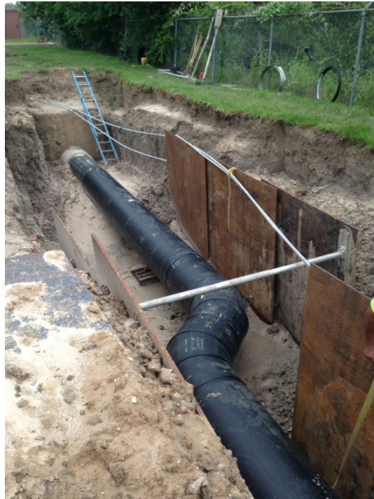
Figure 4: Fused HDPE bends forming one continuous length of pipe.
