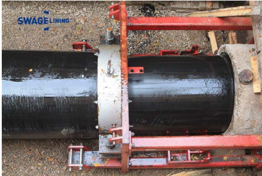
Figure 1: Swagelining™ process as HDPE is pulled through the reduction die.
