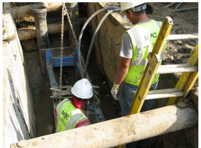
through, the host pipe is split. An expander attached to the tooling forces the fragmented pipe into the surrounding soil while simultaneously pulling in the new pipe.
