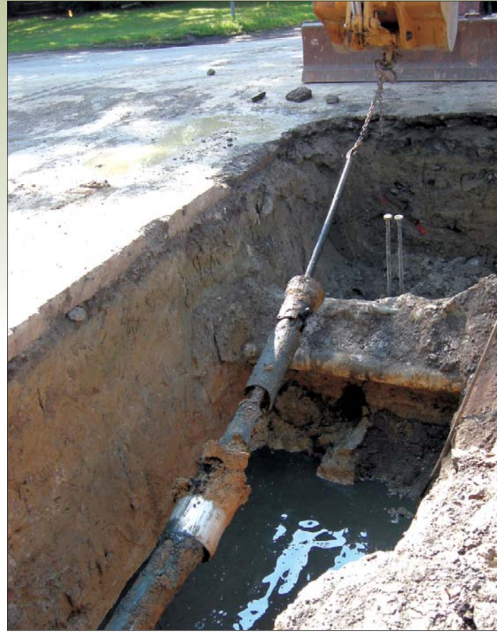
Pre-chlorinated pipe bursting has been approved for use in 36 states.
