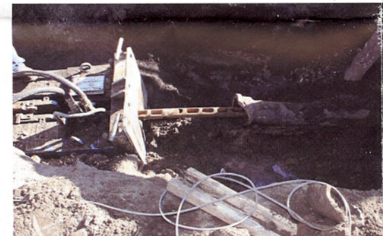
Pipebursting equipment pushes new pipe through the existing bore.
