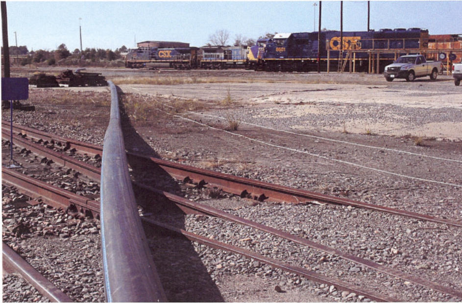
Pipe awaiting installation stretches across tracks southwest of the coach shop.
