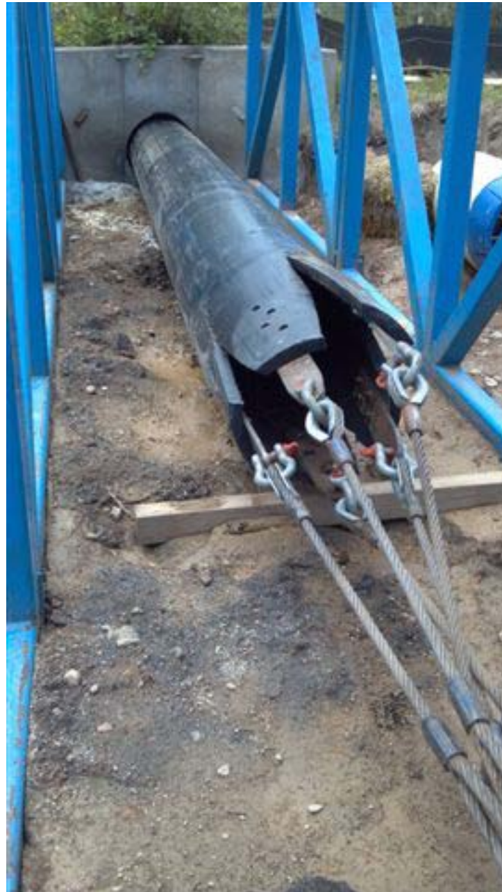
Figure 4: Colorado Swagelining Installation
