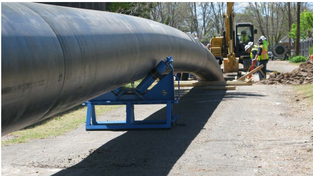
Figure 3: Texas Swagelining Installation
